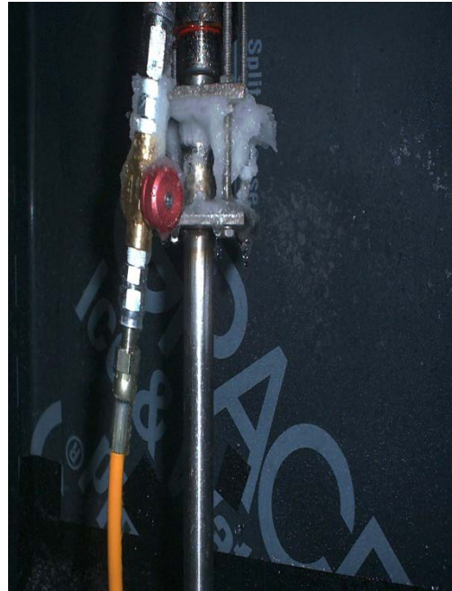
Figure 21. Modified CJHR at Shutdown
